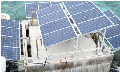
Solar energy street lights on Song Tu Tay islands
