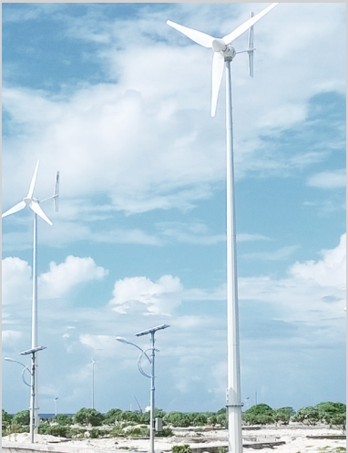
Project Desalination system in Southwest Cay Island (Song Tu Tay). Capacity: 02 wind turbines Xzeres 10kW, 01 wind turbine Skystream 3.7 with 24,4kW in total
